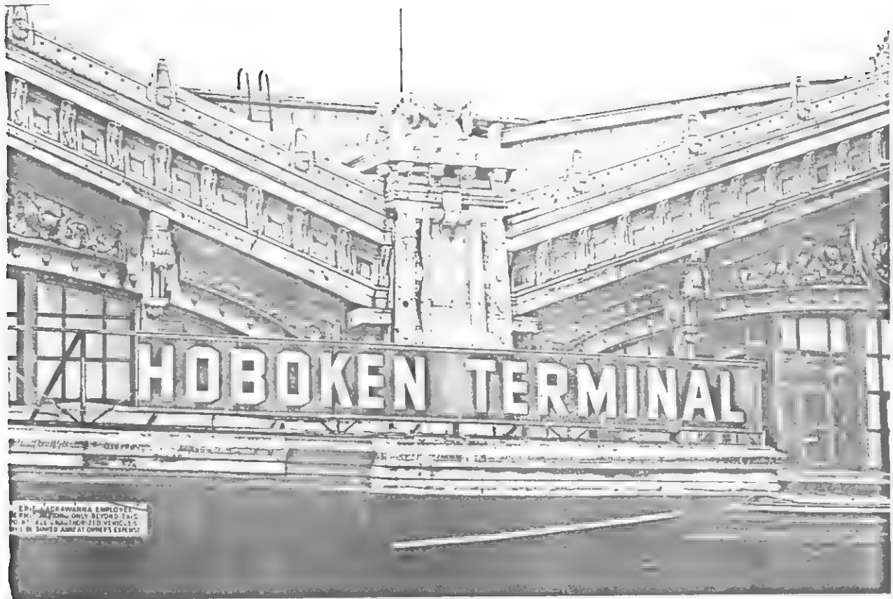
Elliptical, arched windows of ferry terminal building face the terminal's ferry plaza.
